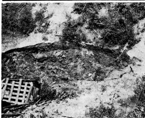
STILL FALLING —Subsidence at top of sealed off slope opening of Fellin mine exemplifies dangerous working conditions under which volunteers labored.
