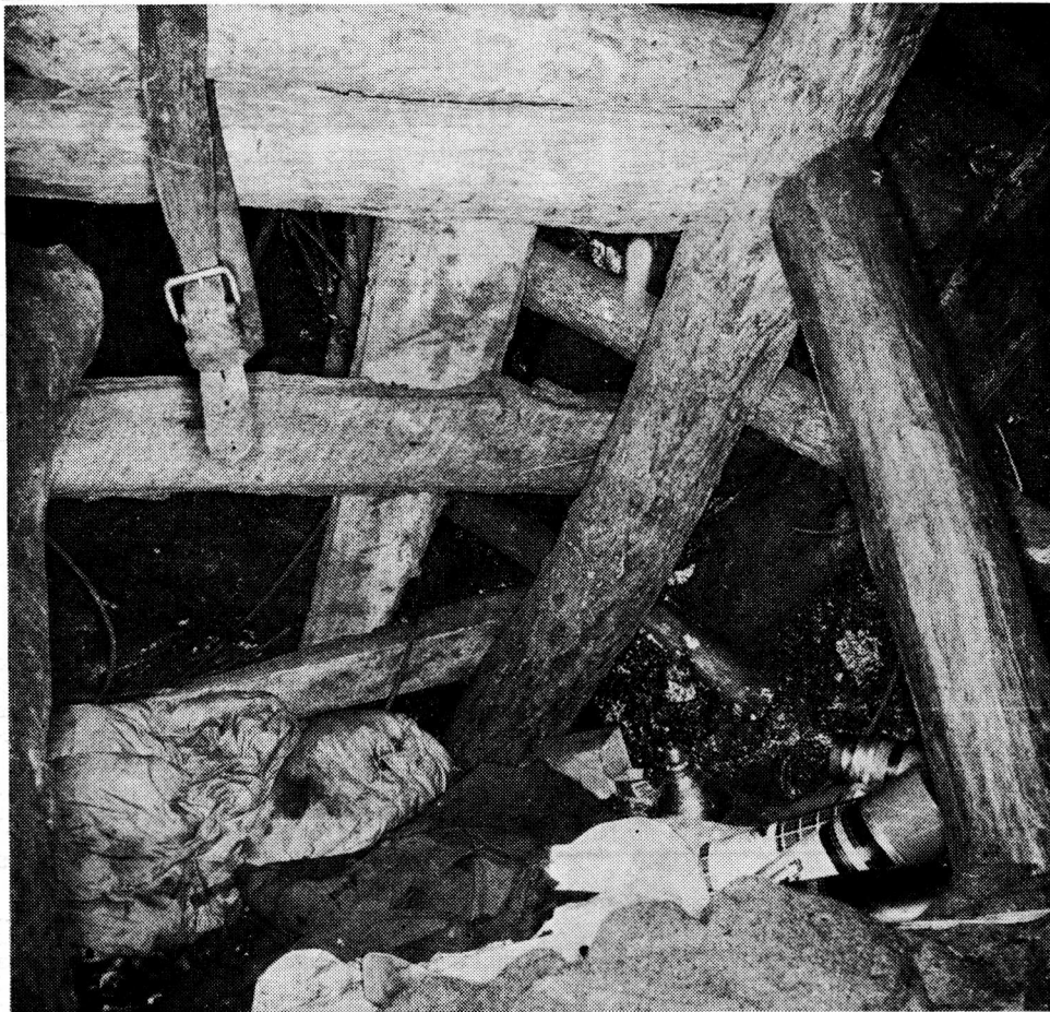
FIRST PUBLIC PICTURE —This is first of two photographs of underground chamber in Fellin mine ever made public. This is a partial view of area in which Fellin and Throne were entombed. Exclusive pictures were taken by Frank Sturges of the Penna. Drilling Company.
